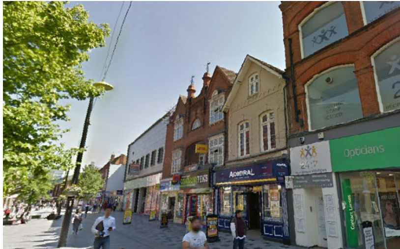
Photograph of 198 High Street (Admiral) and adjoining property
